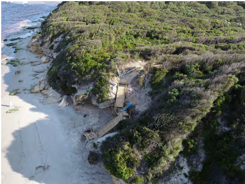
Stairs under construction, Ocean Beach
