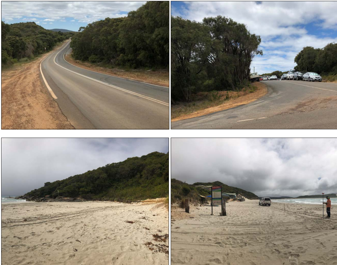
Figure 4: Typical site conditions along Ocean Beach Road (top left), at the entrance of the beach carpark (top right) and along the foreshore on Ocean Beach (bottom left and right).
