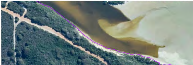
Figure 7-1 Southern embankment of the Inlet (narrow buffers to gravel road)
