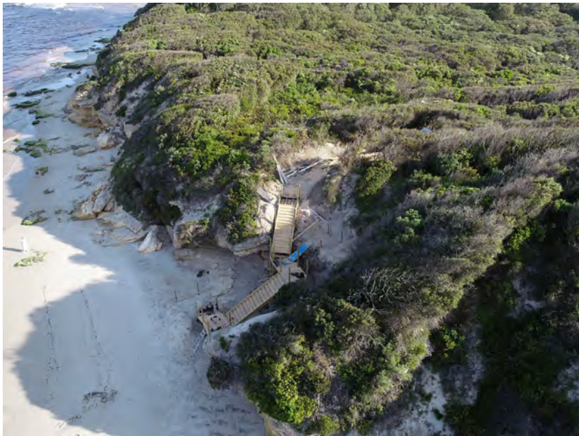
Stairs under construction, Ocean Beach
