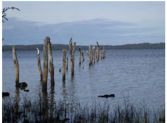
Plate 10 Remnants of the historical jetty
