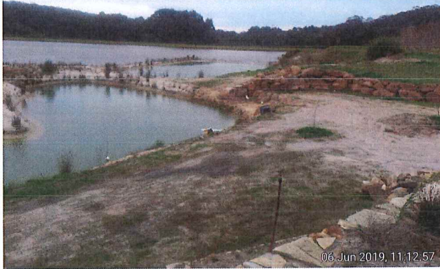
View east from Retreat site across adjoining dams to Wentworth Road along the tree line.
