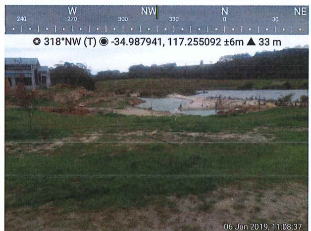
Maintained grass area along entrance road with dams in the background.
