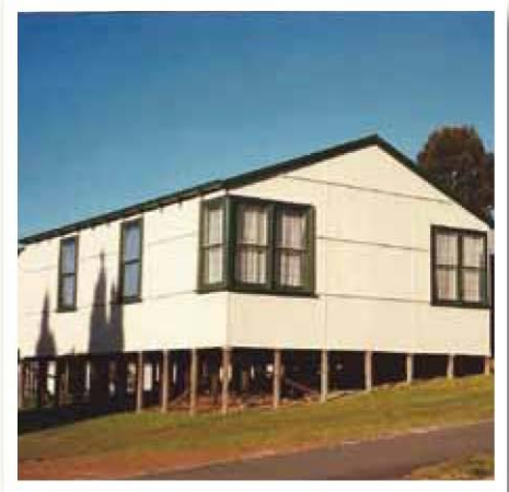
A view of the CWA facilities, showing the prominent hall elevation.
