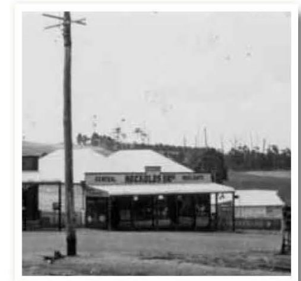
An earlier image of collection of shops along South Coast Highway.
