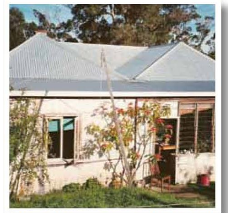
A view of the rear elevation with the double hipped roof.
