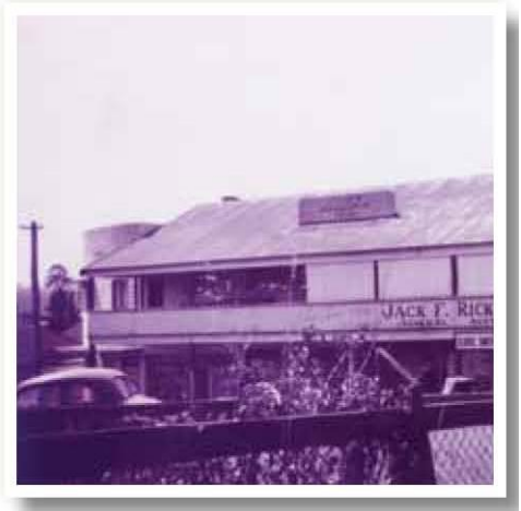
Rear view of the building.
