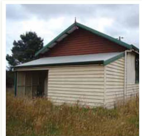
The rear of the hall in 2010.
