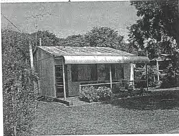
Photo 27 Bullnose verandah is not an authentic detail
