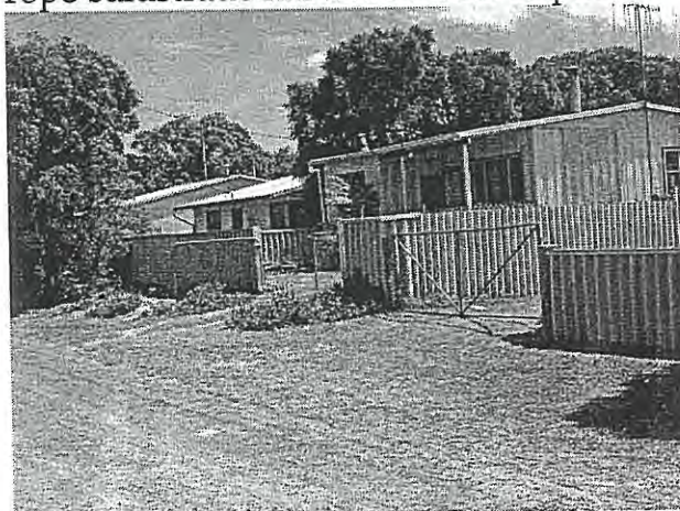
Photo 51 Solid super six fence on Fourth Avenue is visually intrusive
