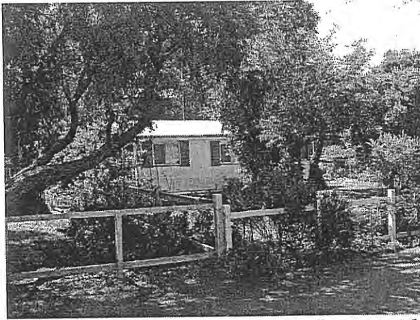
Photo 47 Light post and rail fence with mesh insert has low visual intrusion
