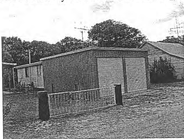
Photo 45 Large steel shed constructed close to the front boundary
