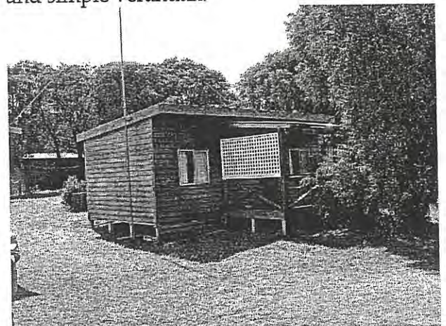
Photo 8 Timber clad skillion The lattice work to the verandah addition is not an authentic detail.
