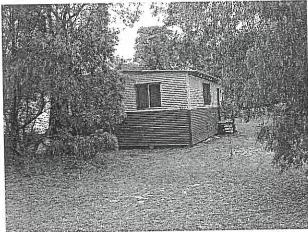
Photo 19 Authentic cladding has been replaced with colorbonded corrugated steel
