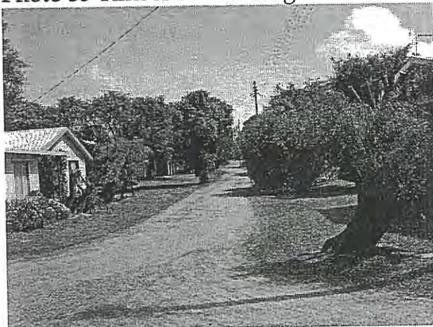
Photo 37 The road form is often curved. Roads curve around pre-existing peppermints. The roads are single lane and paved with gravel. There are no kerbs, drains, signs or other visual clutter.
