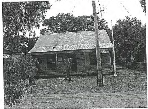
Photo 6 "Shannon" a jarrah clad mill cottage
