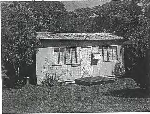
Photo 3 Typical gable cottage
