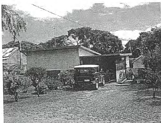
Photo 11 Skillion roofed jarrah and fibro house The simple carport is in keeping with the aesthetic of the precinct.
