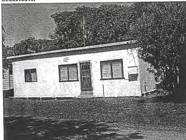
Photo 7 Shallow pitched skillion The room to the left is an addition.
