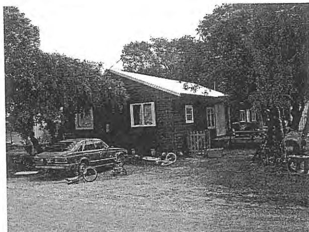
Photo 10 Typical jarrah mill house Appropriately maintained and refurbished. The introduced platform deck is simple and has no decorative elements or balustrading.
