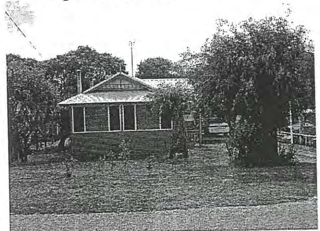
Photo 24 House has recently been extended and reclad with corrugated customorb Decorative elements such as that on the gable are not authentic to the place, neither is the hipped carport.
