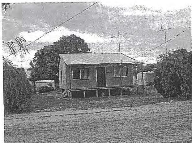
Photo 9 Typical fibro clad gable cottage The verandah has been added.
