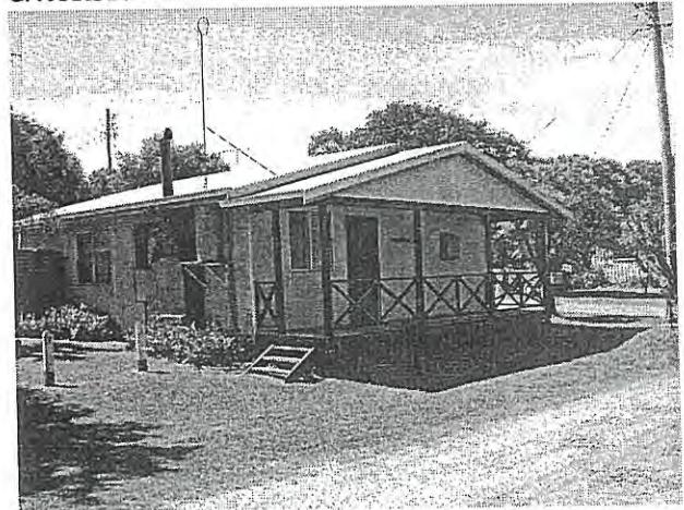
Photo 28 New verandah New verandahs are starting to be added. Decorative elements such as crossed balustrading are not authentic to the precinct.
