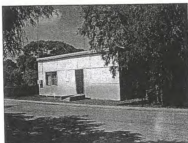
Photo 13 Typical fibro skillion in authentic condition
